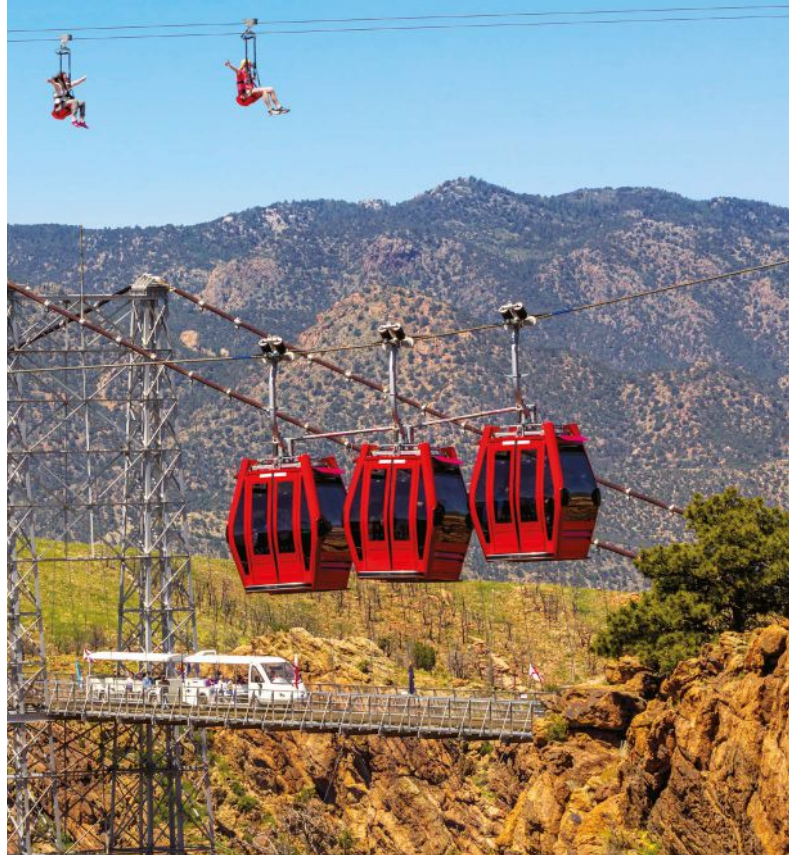
Royal Gorge Bridge & Park
